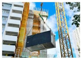
"Chung Yuet Lau" in Jat Min Chuen is built with steel MiC, which helps shorten the duration of superstructure works and reduce construction waste, significantly minimising the impact on nearby residents.
